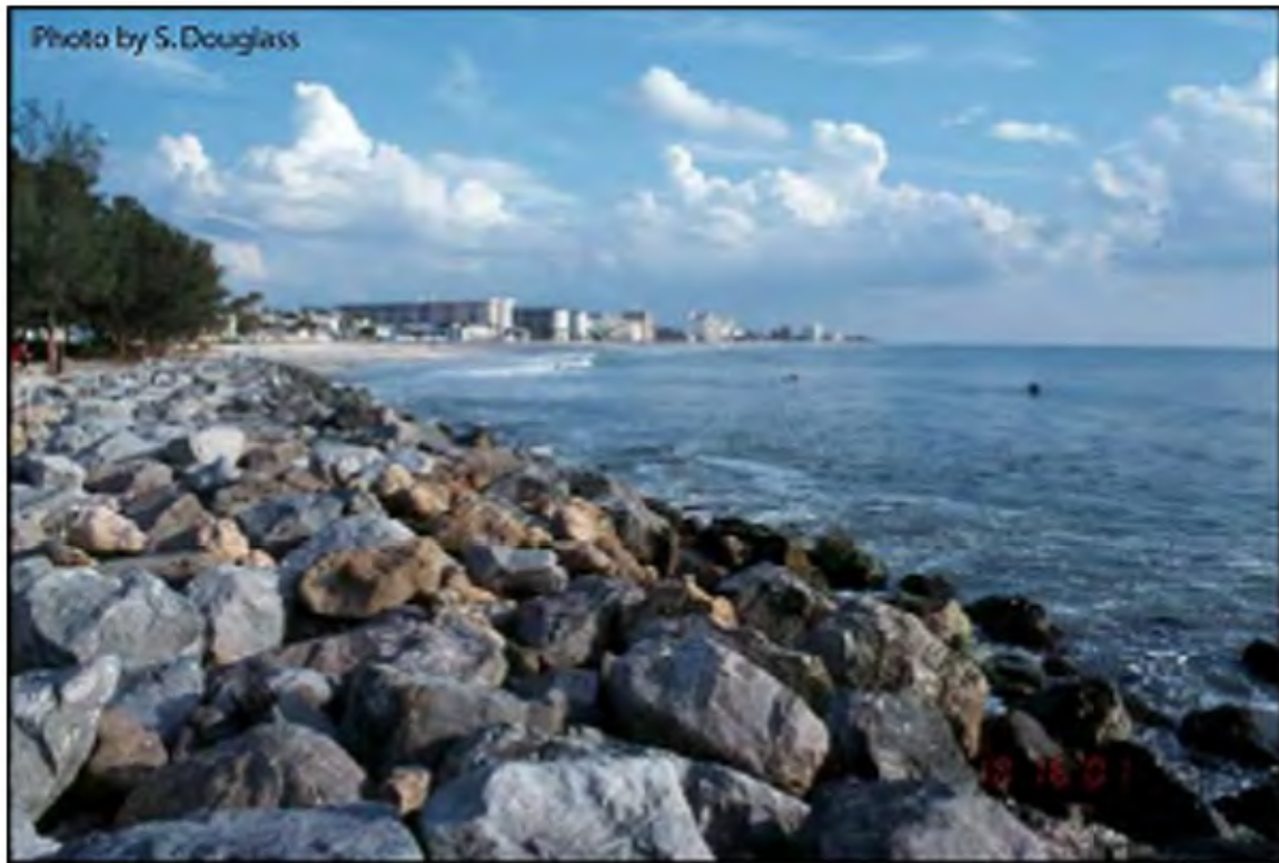
Figure 6.5. Seawall protecting a coastal highway. Venice, Florida (2001)
