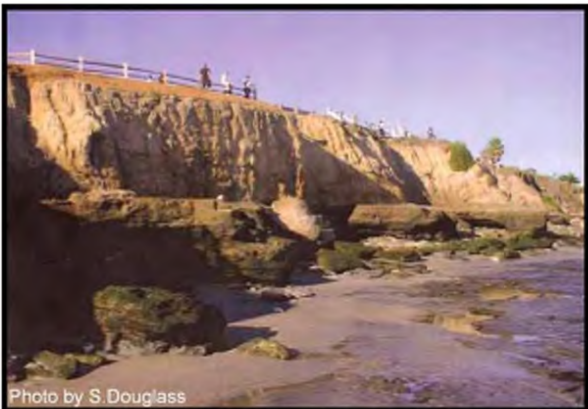
Figure 6.12. Concrete seawall designed to look like the natural rock formation built on an eroding sea cliff to protect a local road. East Cliff Drive, Santa Cruz, California
