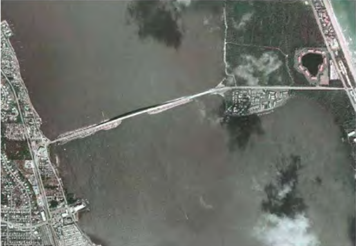
Figure 9.10. Jensen Beach Causeway bridge.
