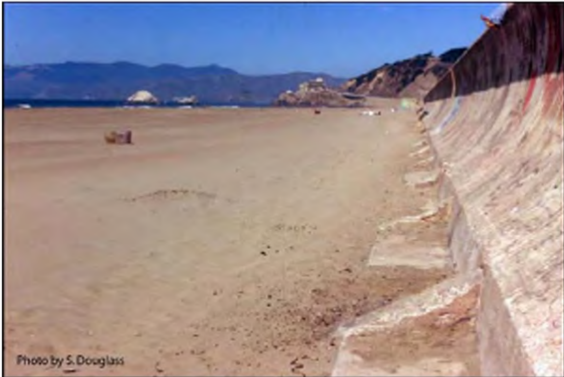
Figure 6.4. San Francisco's Great Highway Seawall. California Highway 35 (1991)
