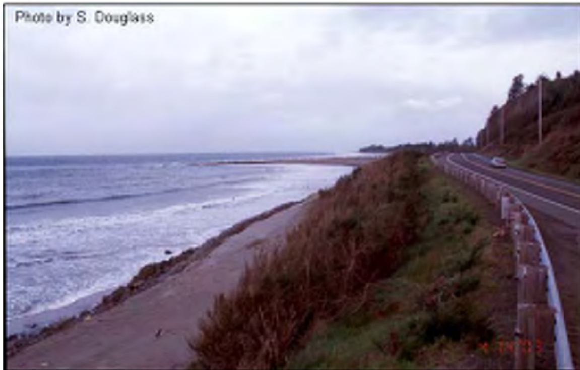
Figure 7.2. A highway initially built inland now threatened by long-term shoreline erosion. Cape Shoalwater area of Washington State Road 105 (2003)
