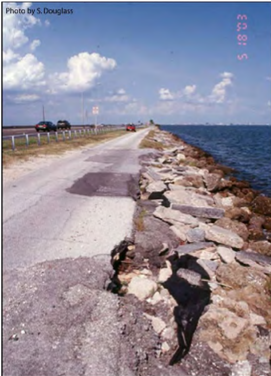
Figure 6.9. Revetment protecting a highway along a bay shoreline. Florida Highway 60, Tampa Bay, Florida (2003)
