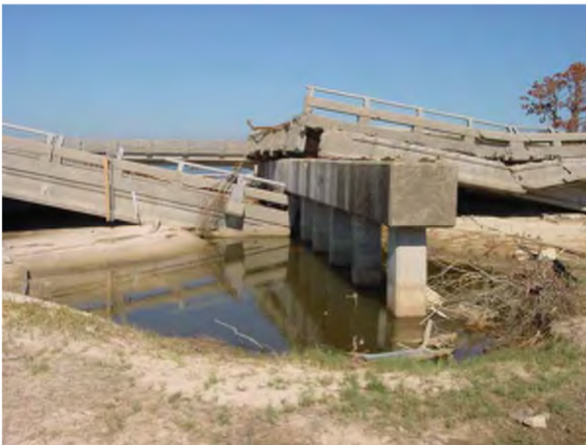
Figure 9.7. Wave scour hole formed by Hurricane Katrina.
