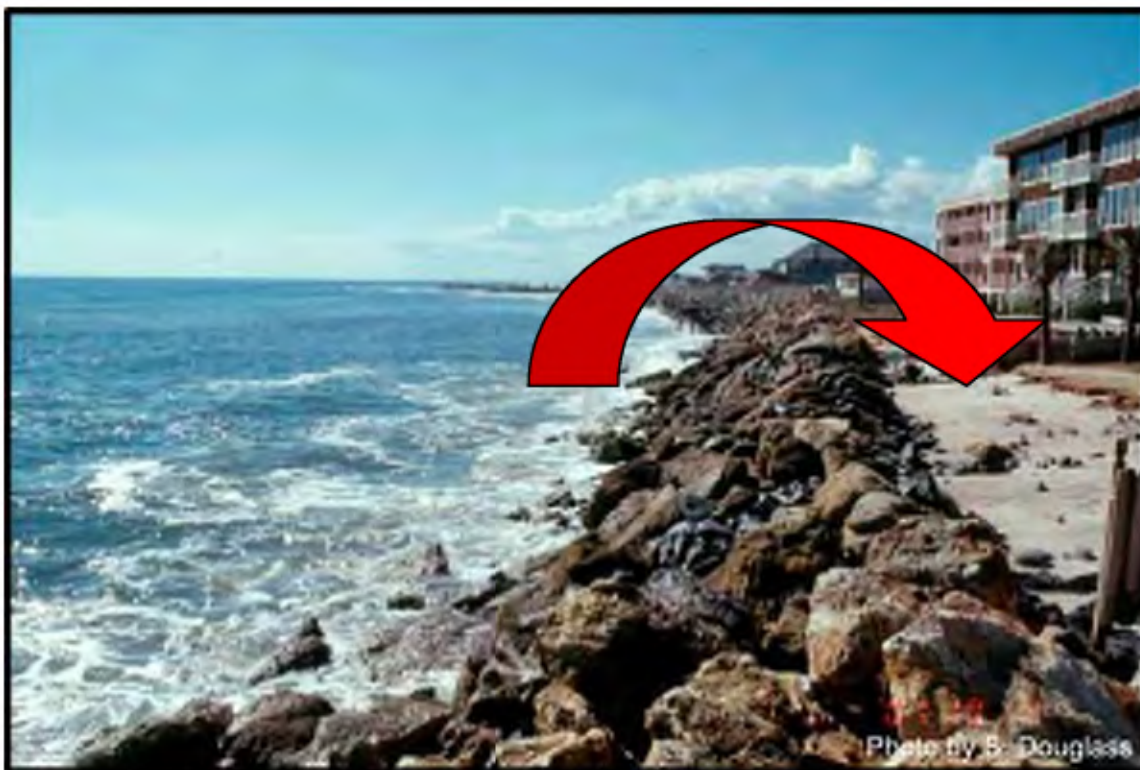
Figure 6.16. An example of splash damage behind seawall
