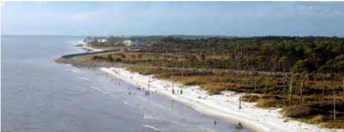
Figure 7.1. A road initially built inland of a receding shoreline is now in the sea. Stump Hole area of Cape San Blas, Florida (2005 FDOT photo)
