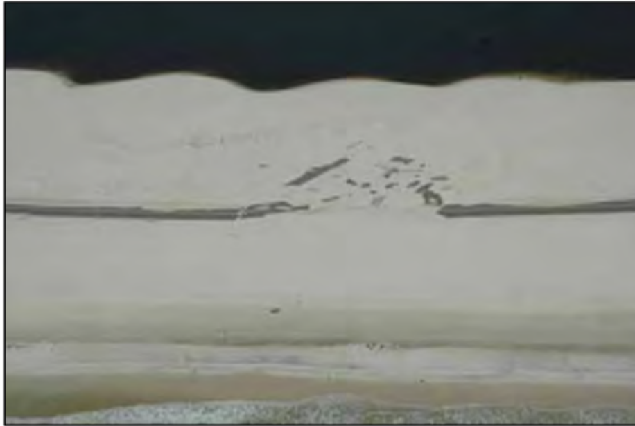
Figure 8.14. Pavement moved landward by overwash processes. (Gulf Islands National Seashore, Perdido Key, Florida after Hurricane Ivan; 2004).
