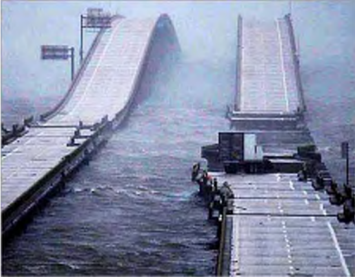
Figure 9.13. Interstate-10 bridge across Escambia Bay, Florida, after Hurricane Ivan. Photo looking east from Pensacola at dawn September 16, 2004. (Pensacola News Journal photo)
