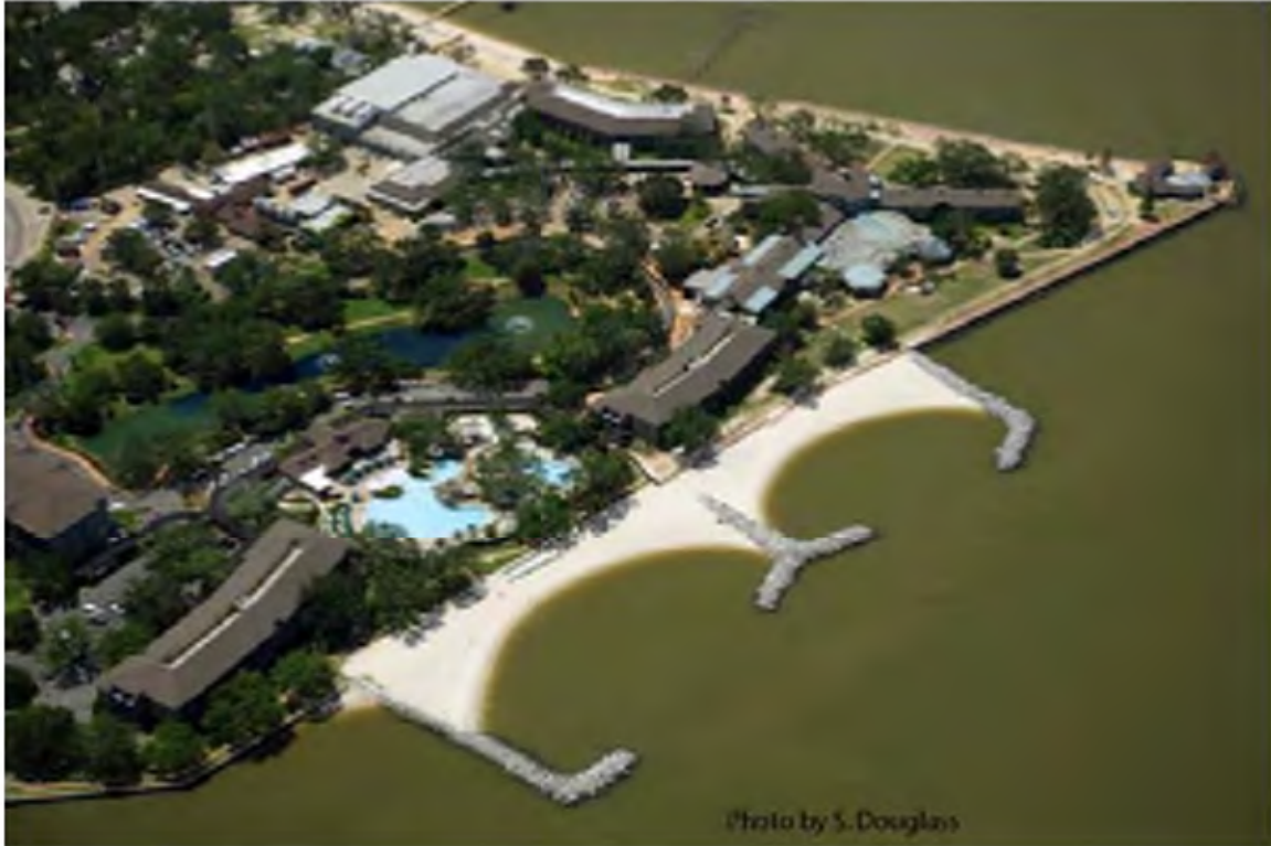
Figure 7.23. Constructed pocket beach stabilized with a T-head groin breakwater system (Point Clear, Alabama).
