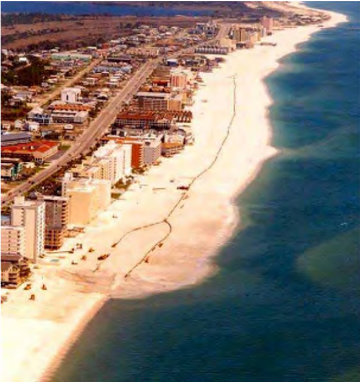
Figure 7.15. A beach nourishment project under construction. Gulf Shores, Alabama (2001)
