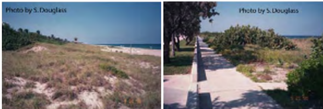
Figure 7.16. Beach nourishment project with constructed dune on top of old, failed revetment protecting road. Florida Highway A1A, Delray Beach (2001)
