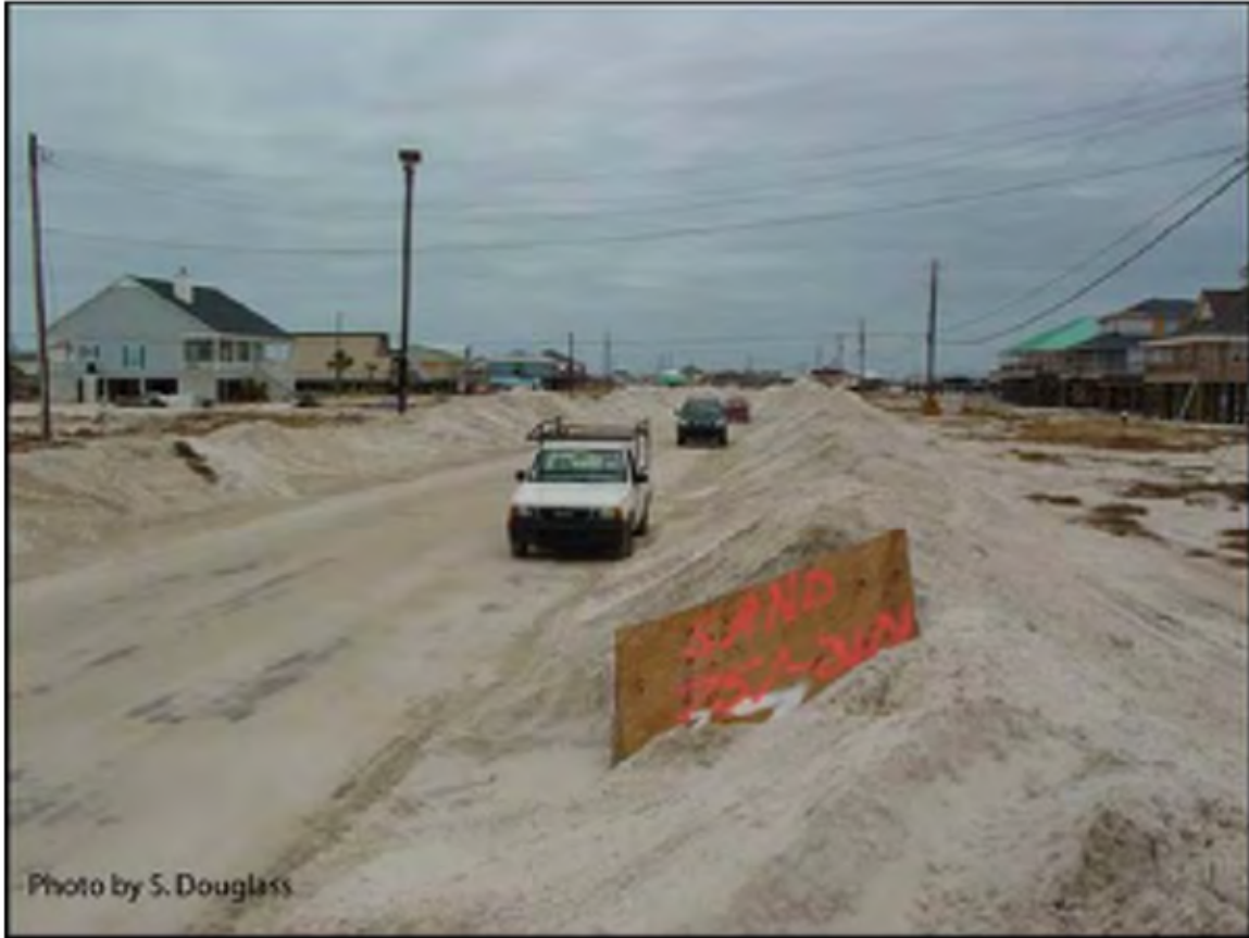
Figure 8.17. Example of road buried by overwash and opened by plowing sand off
